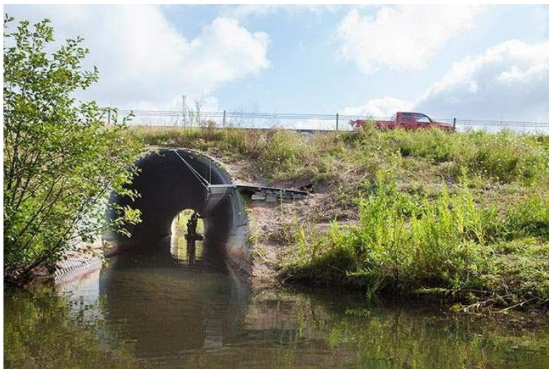
Figure 4. Examples of dry passageways created for small- and mid-sized mammals (USDA, NYSDOT, TNC).
