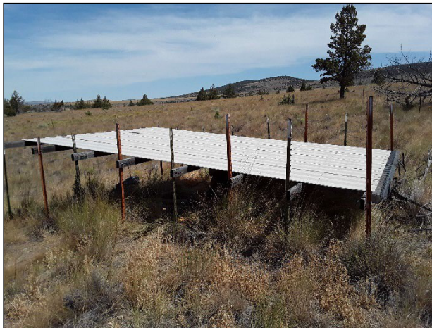
Figures 1 and 2 above display a few of the parts that make up a guzzler; a rainwater catchment apron with storage tank underneath, as well as a drinking basin.
