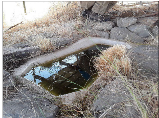
Figures 1 and 2 above display a few of the parts that make up a guzzler; a rainwater catchment apron with storage tank underneath, as well as a drinking basin.
